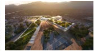
Jury Yulong Snow Mountain Vistor Center Studio 21@CCDI Group
