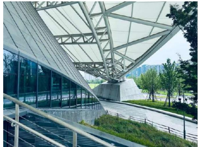
Hockey stadium exterior
