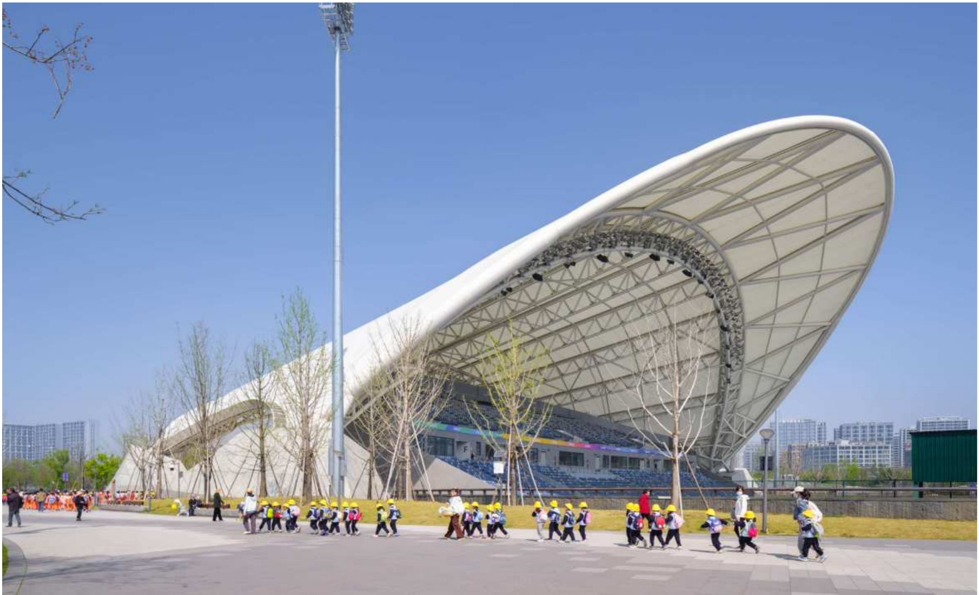
Field Hockey Stadium: The concrete blocks tie the structure to the ground to keep the roof in tension, actually holding it down rather than keeping it up.
